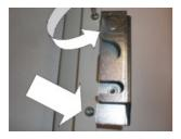
Both Allen screws have to be unscrewed to remove the lock plate. The lock plate can then be removed from the frame profile. Assembly of the new part is performed in reverse disassembly sequence.
