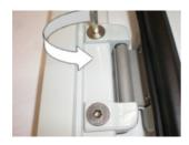
First, the bottom hinge cover has to be disassembled as described under **2.6 Replacement of hinge cover**. Then the hinge eyelets are disassembled as shown in the image. Following this, the hinge is disassembled on the door leaf side as demonstrated in the image to the right under **1.5 Replacement of the window hinge**. Assembly of the new part is performed in reverse disassembly sequence.
